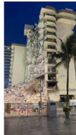
Champlain Towers in Surfside, Fla., collapsed on June 24, 2021. The destruction resulted in the death of 98 residents.
